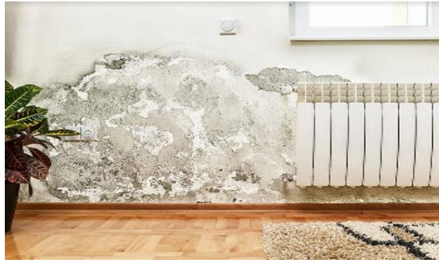
Waterproofing of sunken areas: Bathrooms, toilets, balconies etc
